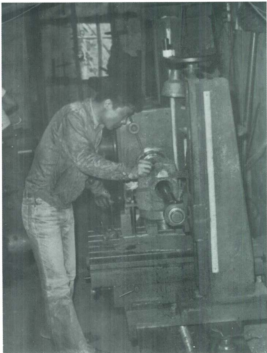
Operating a boring machine in a small-scale factory
